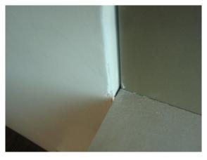
Figure 65: The gap in the same wall shown in Figure 64, where the wall meets the window
